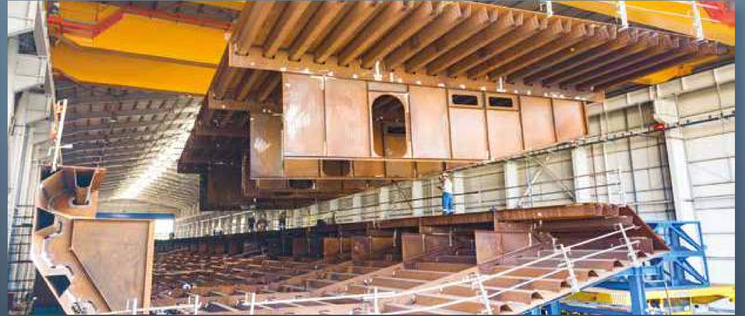
GIRDER BLOCK FORMATION
