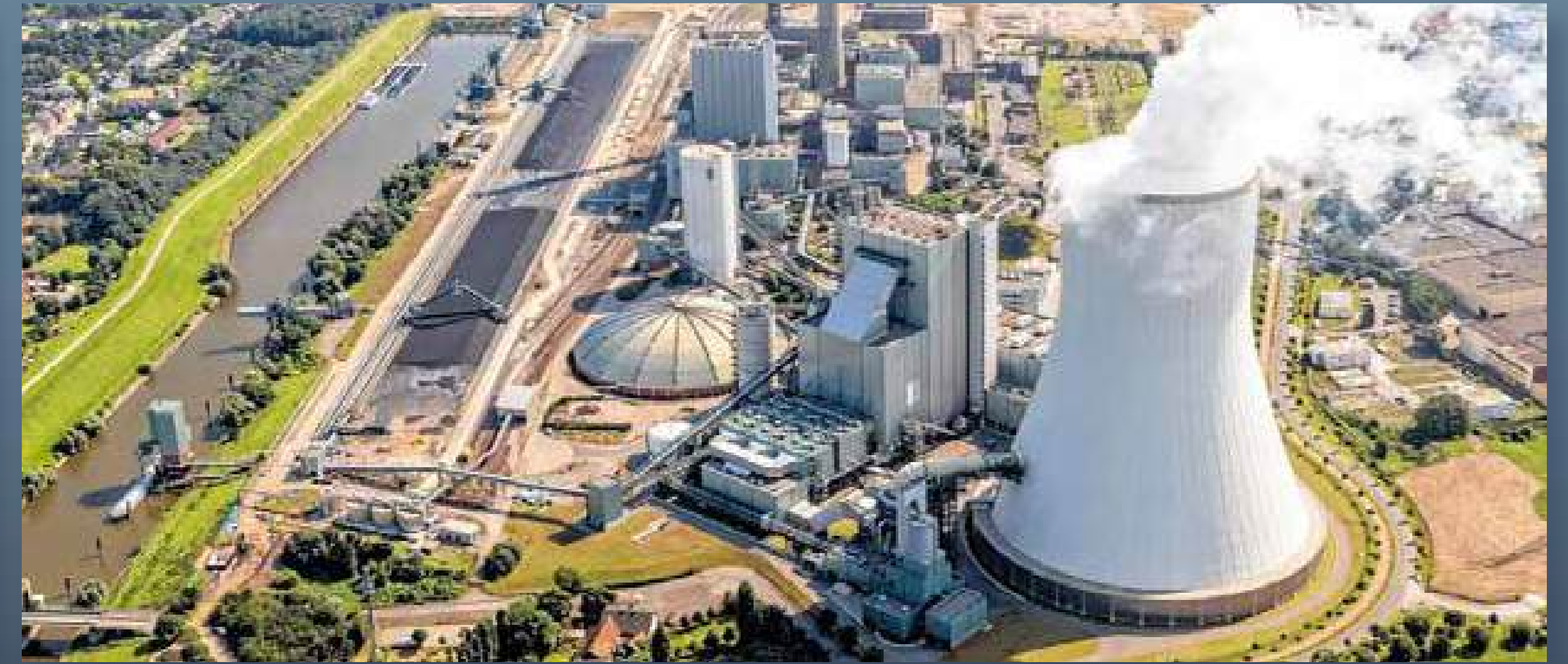
WALSUM COAL FIRED POWER PLANT 800 MW
