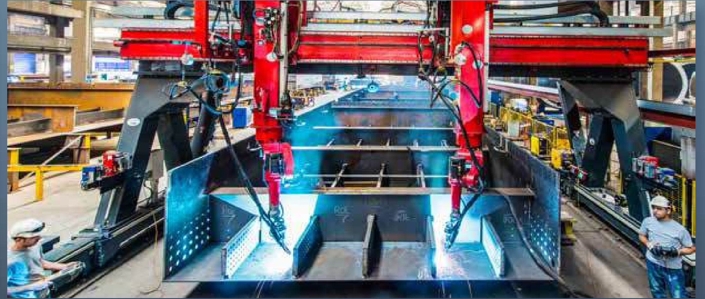
TOWER PANEL FABRICATION
